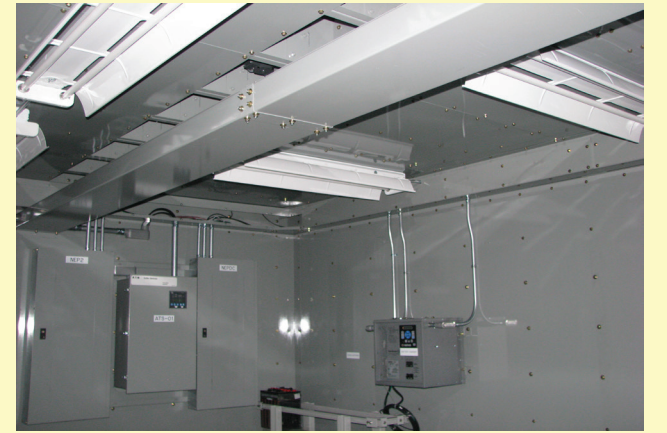
Enclosures can hang 1,000 lb. CPT epoxy copper bus – stand offs as specified – custom boots – wireways for total access
