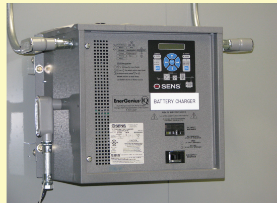
Every option for batteries including seismic - superb signage
