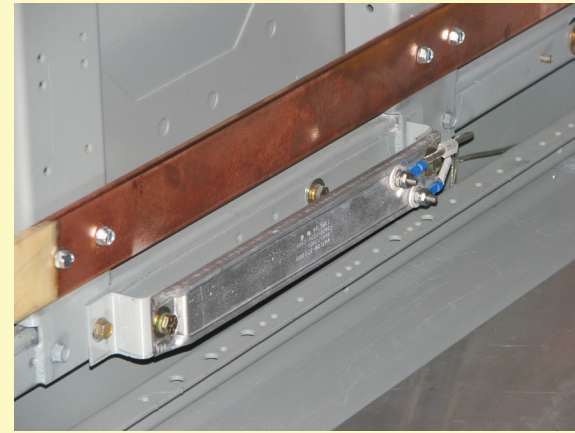
Enclosures can hang 1,000 lb. CPT epoxy copper bus – stand offs as specified – custom boots – wireways for total access
