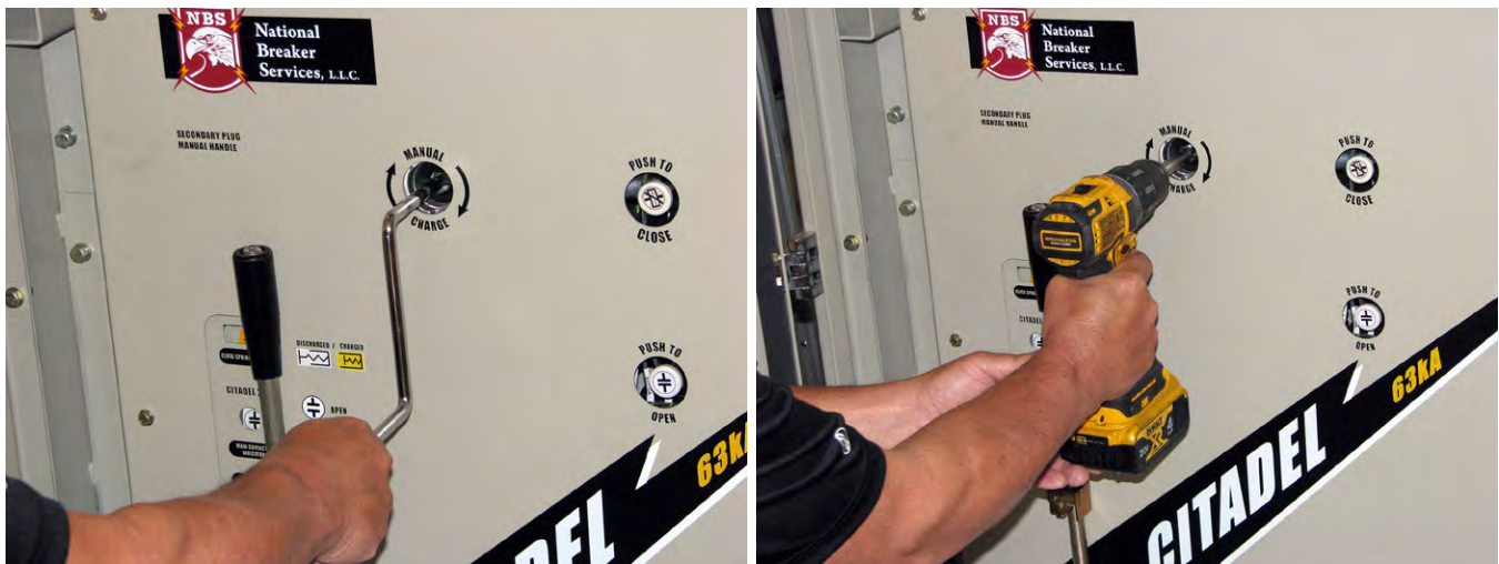
FIGURE 2: MANUAL CHARGING OF CLOSING SPRING
