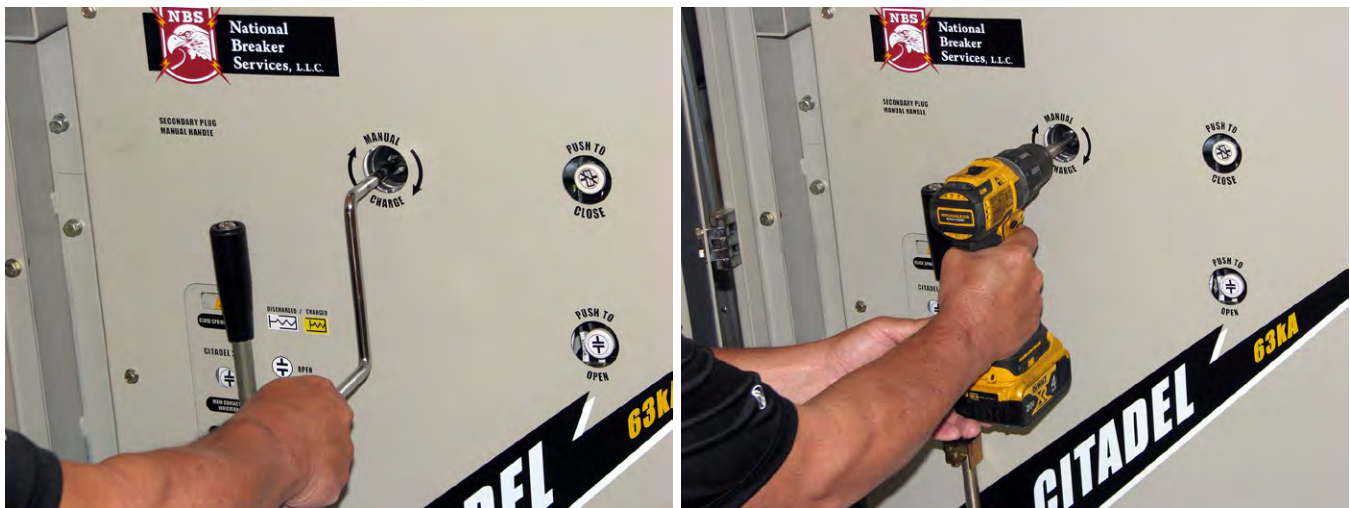
FIGURE 2: MANUAL CHARGING OF CLOSING SPRING
