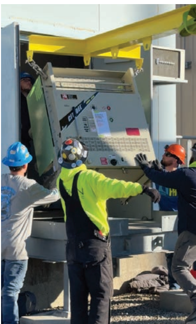
12. Citadel draw-out breaker is introduced to the GAC and its one-high enclosure
