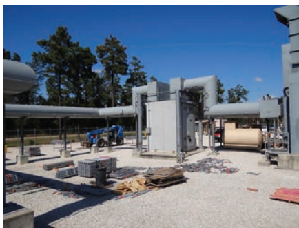
2. Circular non-seg bus runs from the generator (extreme right) to the circuit breaker in the generator accessory cabinet at the center of the left-hand photo; it is shown entering the generator step-up transformer in the right-hand photo
