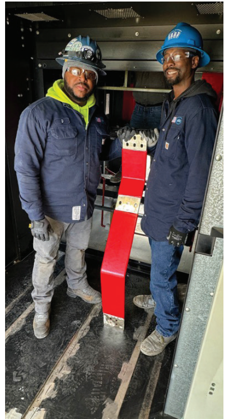
6. Cell fully prepped to receive the retro-fill-kit components
