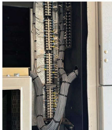
11. Proper wiring connections is a critical step in the retrofit process
