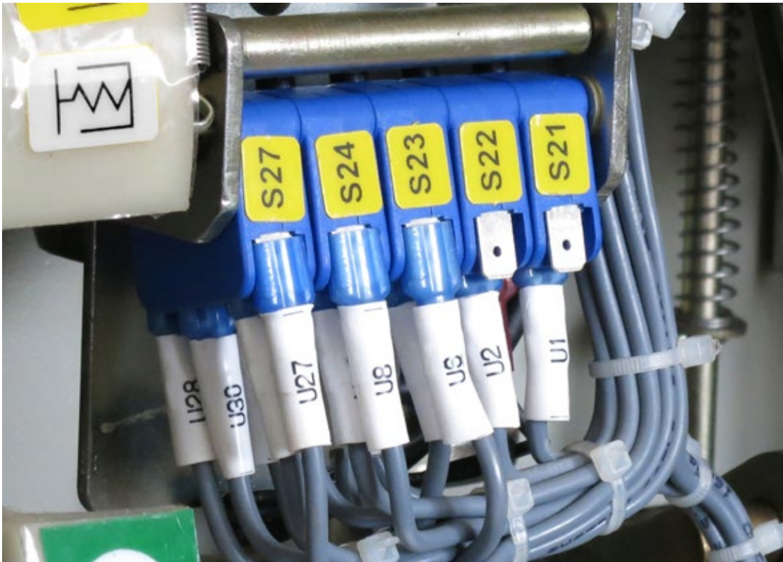
Micro-Switches associated with closing spring:
