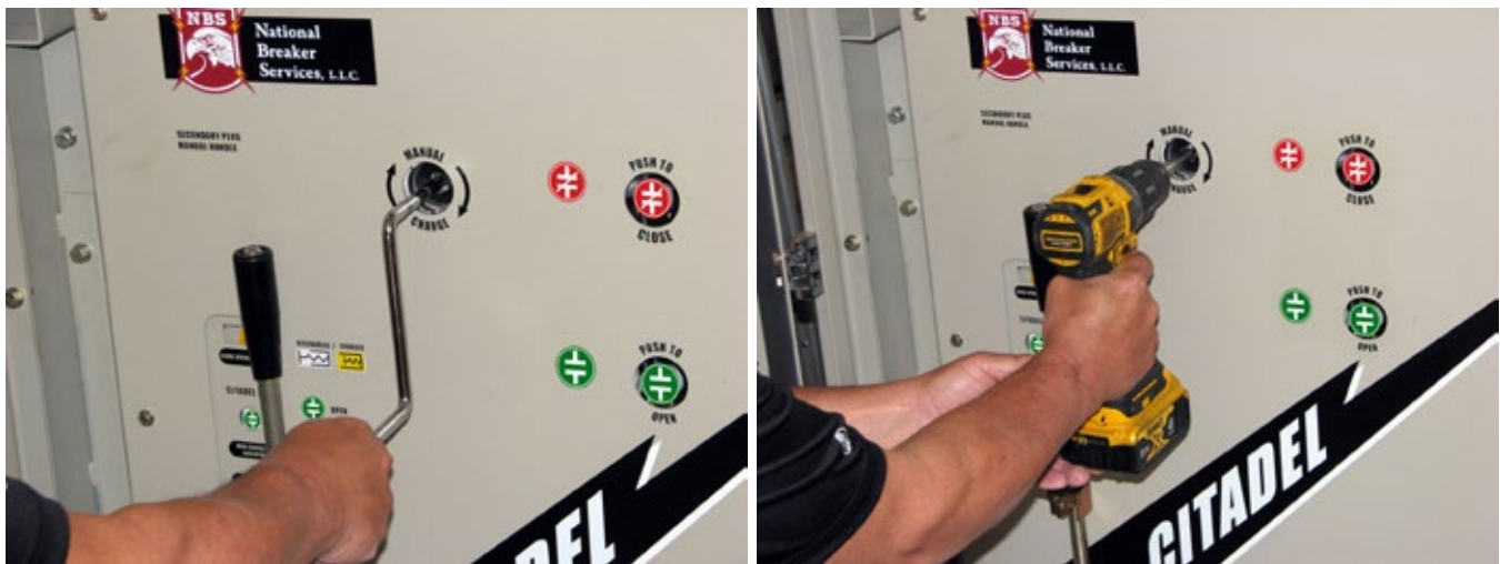
FIGURE 2: MANUAL CHARGING OF CLOSING
