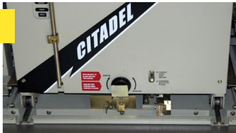
Locked in disconnect position
